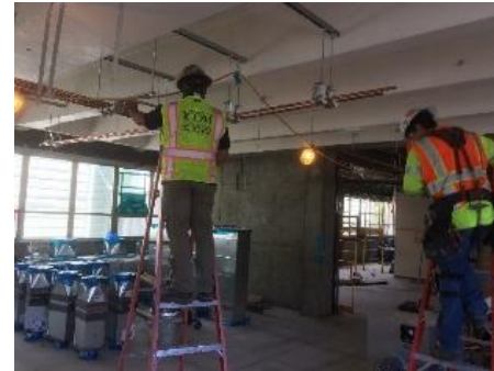
Maxine Hall – MEP installation
